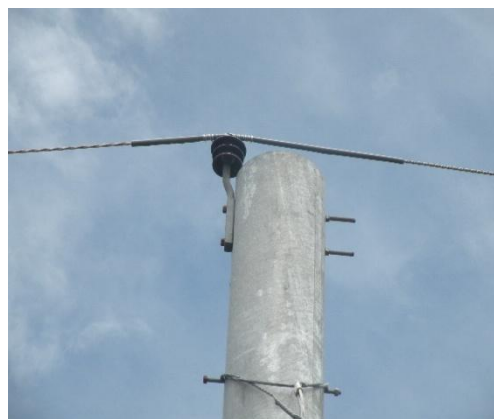
Figure 5: Picture showing example of use of the Overhead Line Cover
